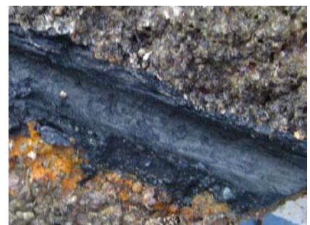
Anaerobic marine corrosion of reinforcing bar recovered from 65-year-old concrete structure.
